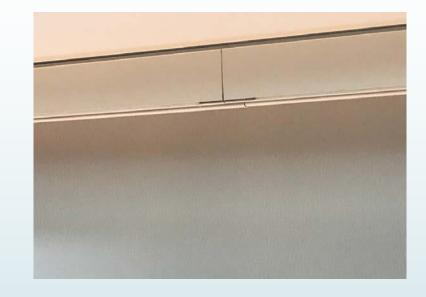
Insert a flat screwdriver into the track groove and push the pins with a hammer towards the other track
